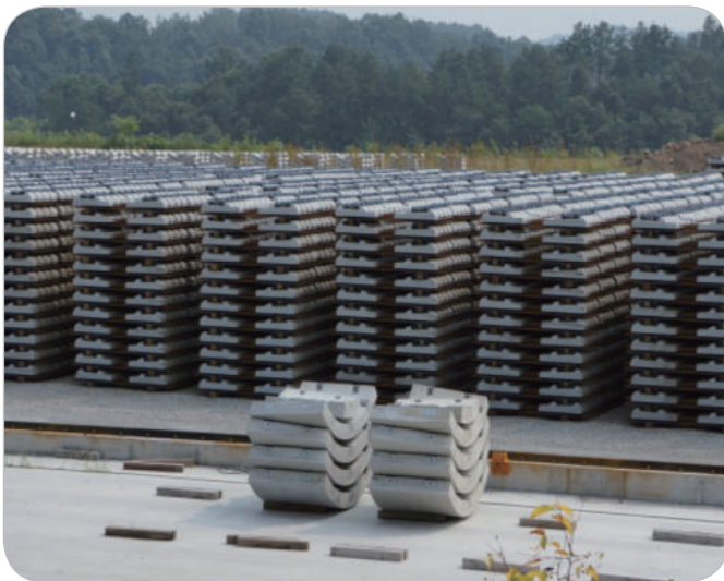
Precast Segments for Tunnel
