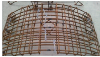
Rebar reinforced segment cage
