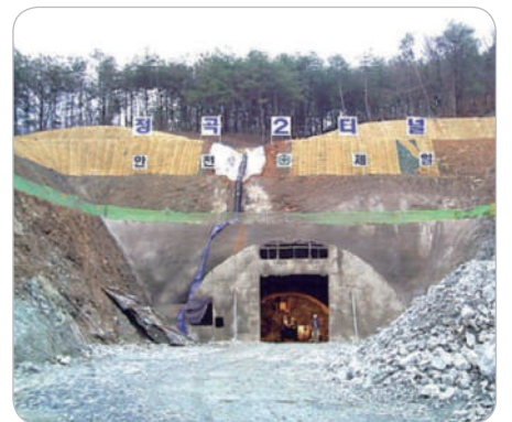
Jeongok Tunnel No. 2
