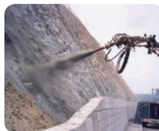
Ground & Rock Support
