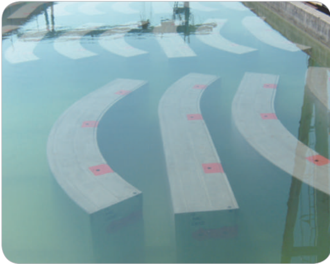
Segment at Curing Stage
