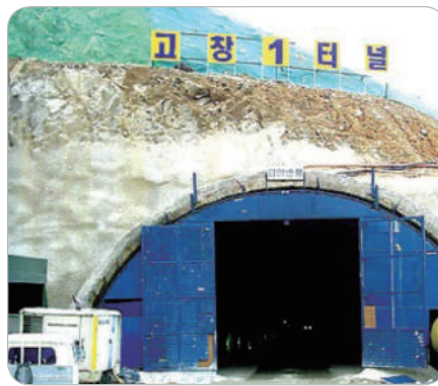
Gochang Tunnel No. 1
