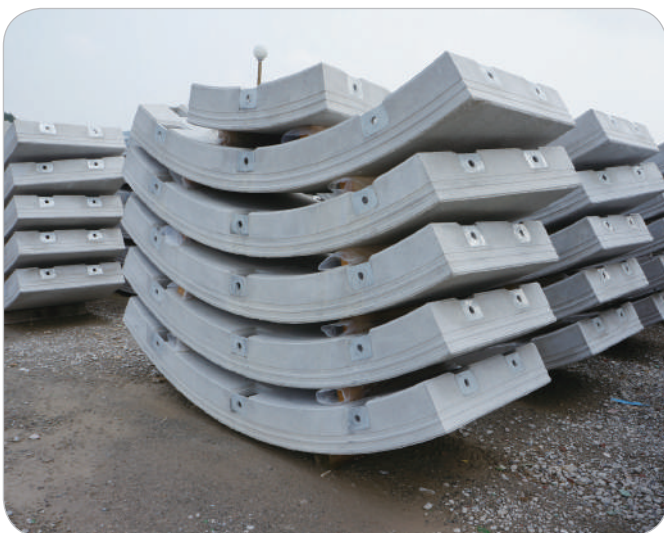
Precast Segments for Tunnel
